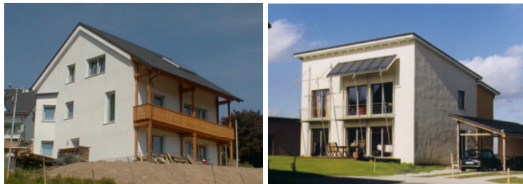
Fig. 2: Object 3 (left): The building in Wenden-Hillmicke, Germany, is a two-family house from pre-built concrete elements with two upper floors and heated basement.
