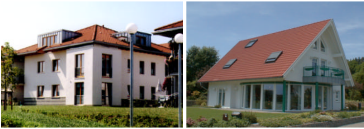
Fig. 1: Object 1 (left): The building in Essen-Kraienbruch, Germany, is a three story multi-family house in massive construction with basement.
